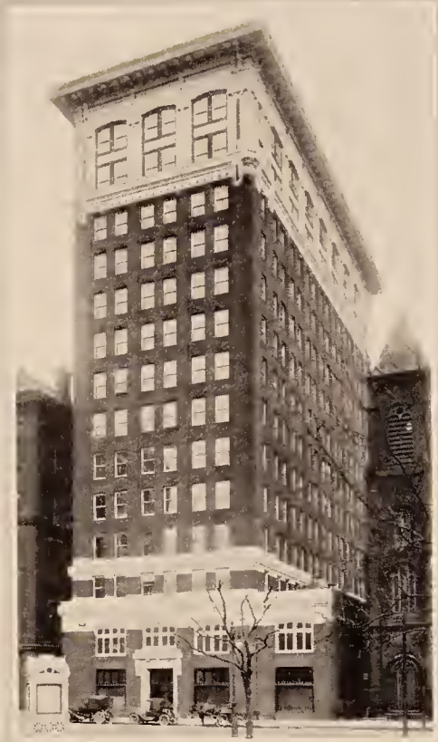
Cleve. Electric Ill. Co. Building
